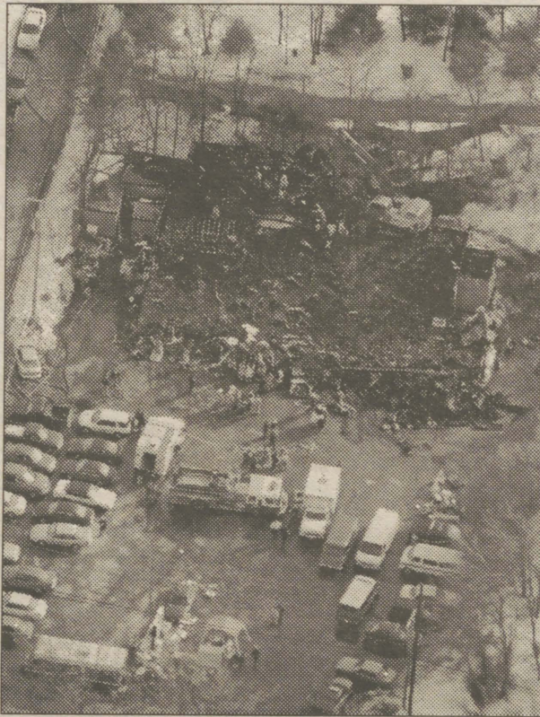
Steve Szydlowski -KRT Workers sort through debris Friday, Feb. 21, at a nightclub where a fire killed dozens and injured more than 150.
