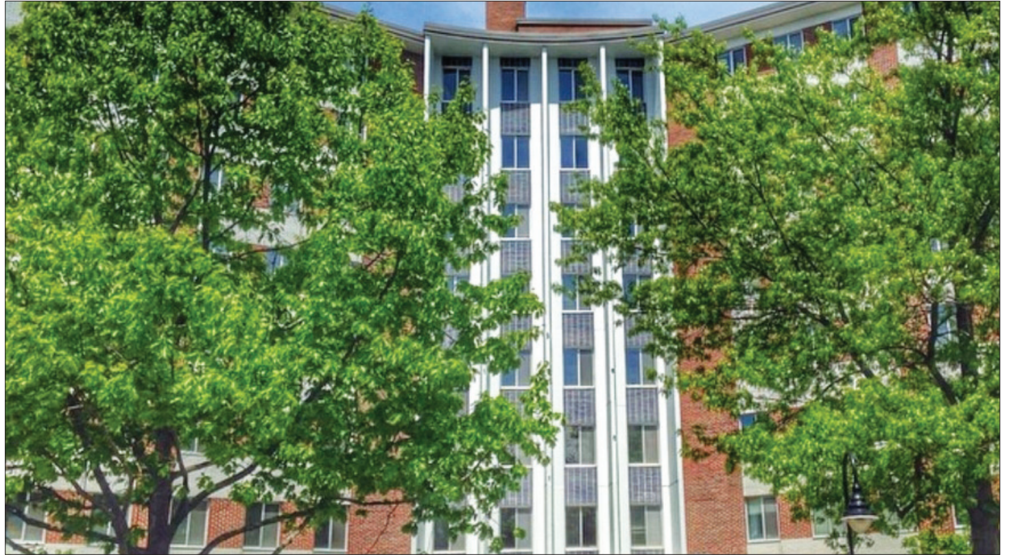
Photo courtesy of the University of New Hampshire
