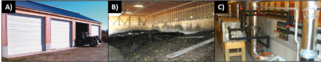
Figure 1. Photos of the Joshua Nelson Energy Recovery Compost Facility. The images show A) the exterior of the facility where compost feedstock is loaded, B) piles of composting material in the facility, and C) the back of the facility where the compost exhaust gas is piped. Sources for images: UNH 2014; Personal communication, Matthew Smith, 2016.
