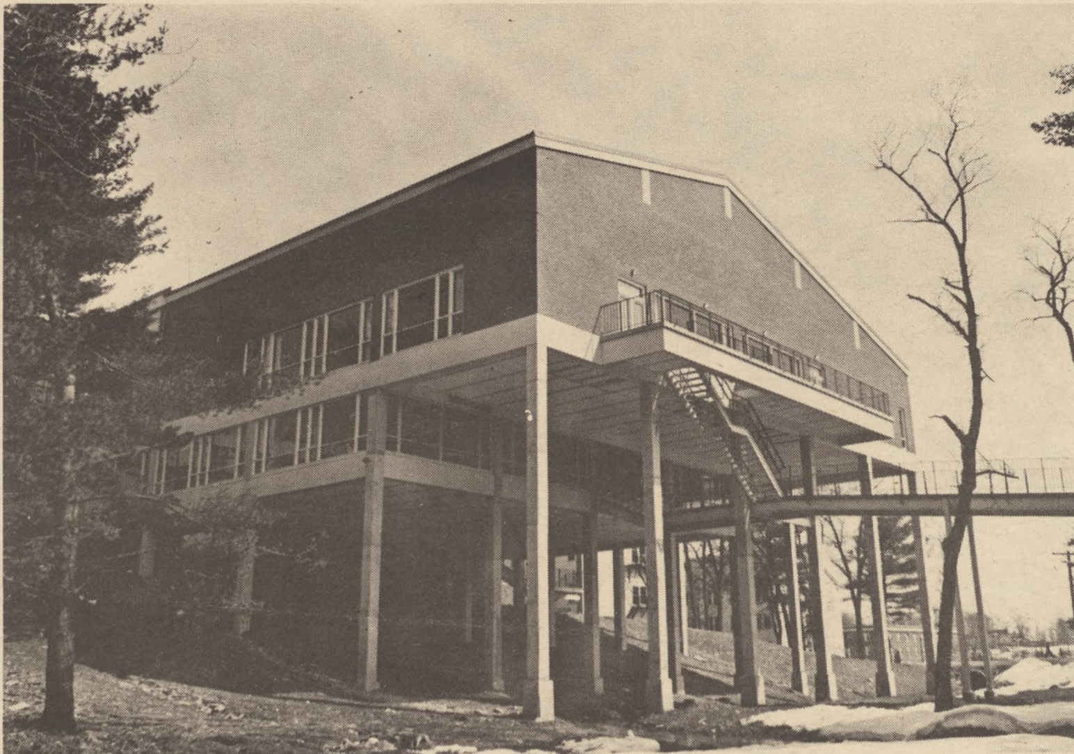
The $1¼ million addition to the Union.
