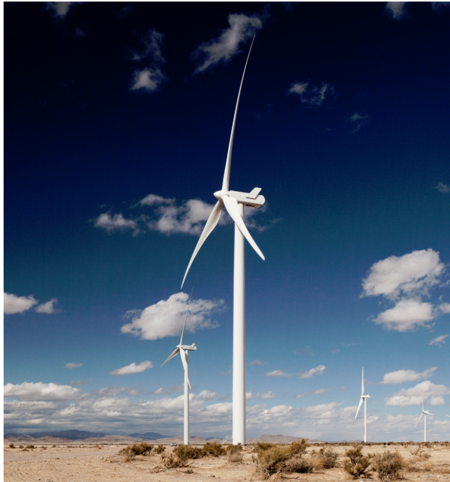
Figure 1.2: Vestas V100 1.8 MW three-bladed axial-flow, a.k.a horizontal-axis wind turbine. Courtesy of Vestas Wind Systems A/S.
