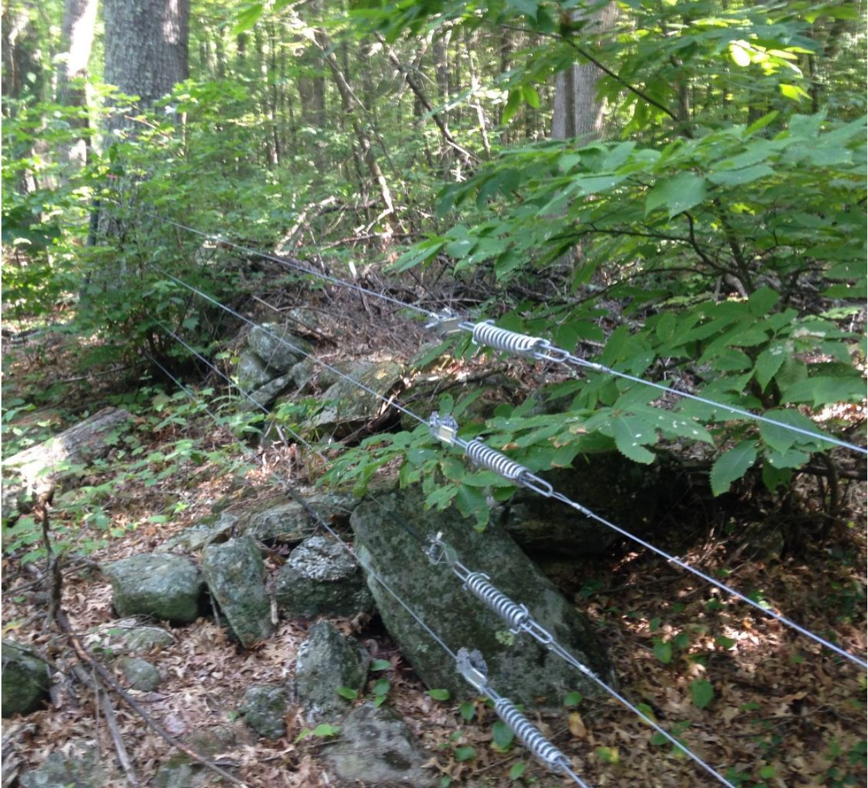
Image 2: Compression springs incorporated into high tensile electric fencing around a new Northeast silvopasture. These springs allow the fence to flex and recover during damage from falling trees or limbs. Additionally, compression springs allow the fence to stretch as tree stems move during wind events.
