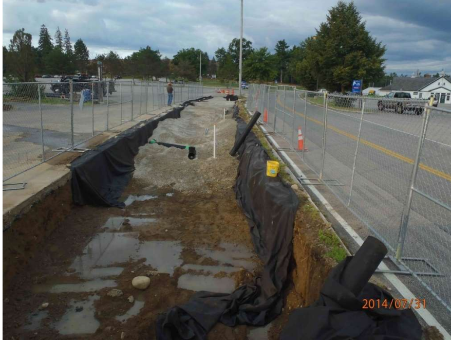
Figure 5: A Lot Gravel Trench Construction after rain
