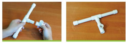
**Step 5:** Insert one end of a 12" pipe piece into the other end of the PVC tee connector.
