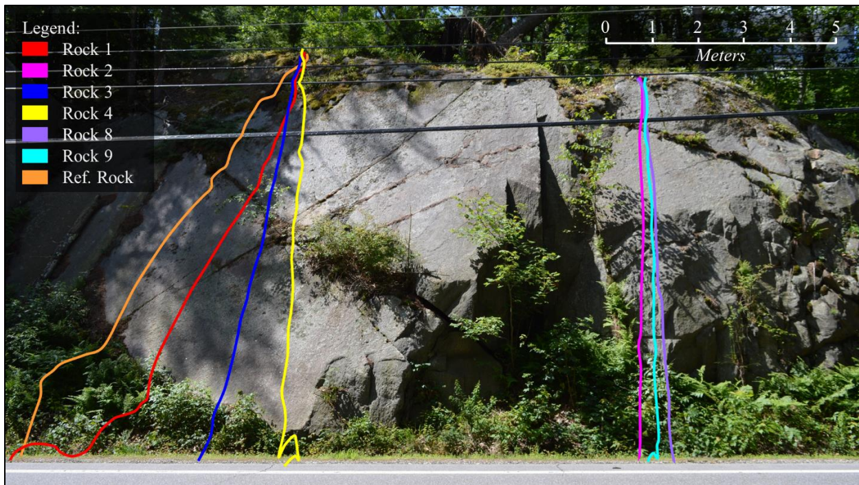
Figure 5.33. Rockfall trajectories: Franklin 2 NH.
