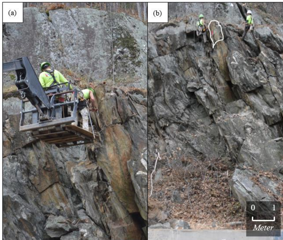
Figure 5.71. First scaled rock (a) during preparation, and (b) before scaling (the pink dot marks the SR location).
