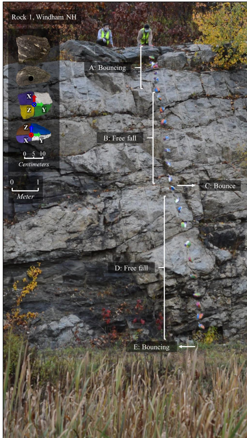
Figure B.88. Rockfall trajectory: rock 1, Windham NH.
