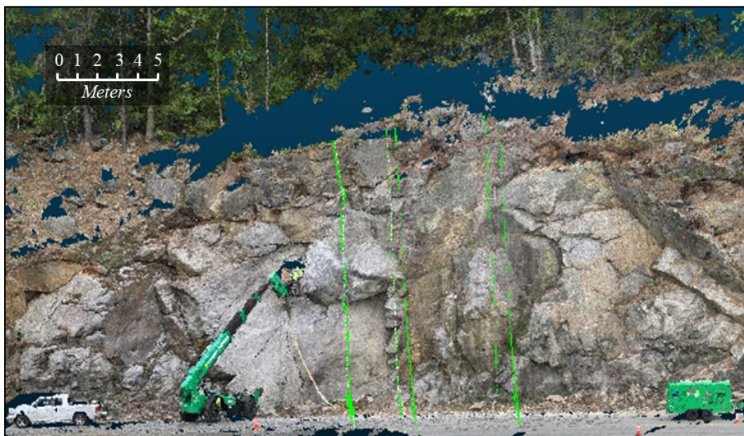
Figure 3.15. 3D point cloud generated by photogrammetry for a test slope in Warner, NH. The green lines represent the cross-section locations for 2D rockfall modeling.
