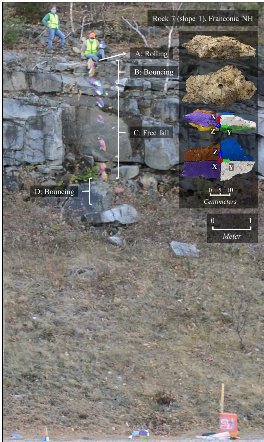
Figure B.23. Rockfall trajectory: rock 7 (slope 1), Franconia NH.
