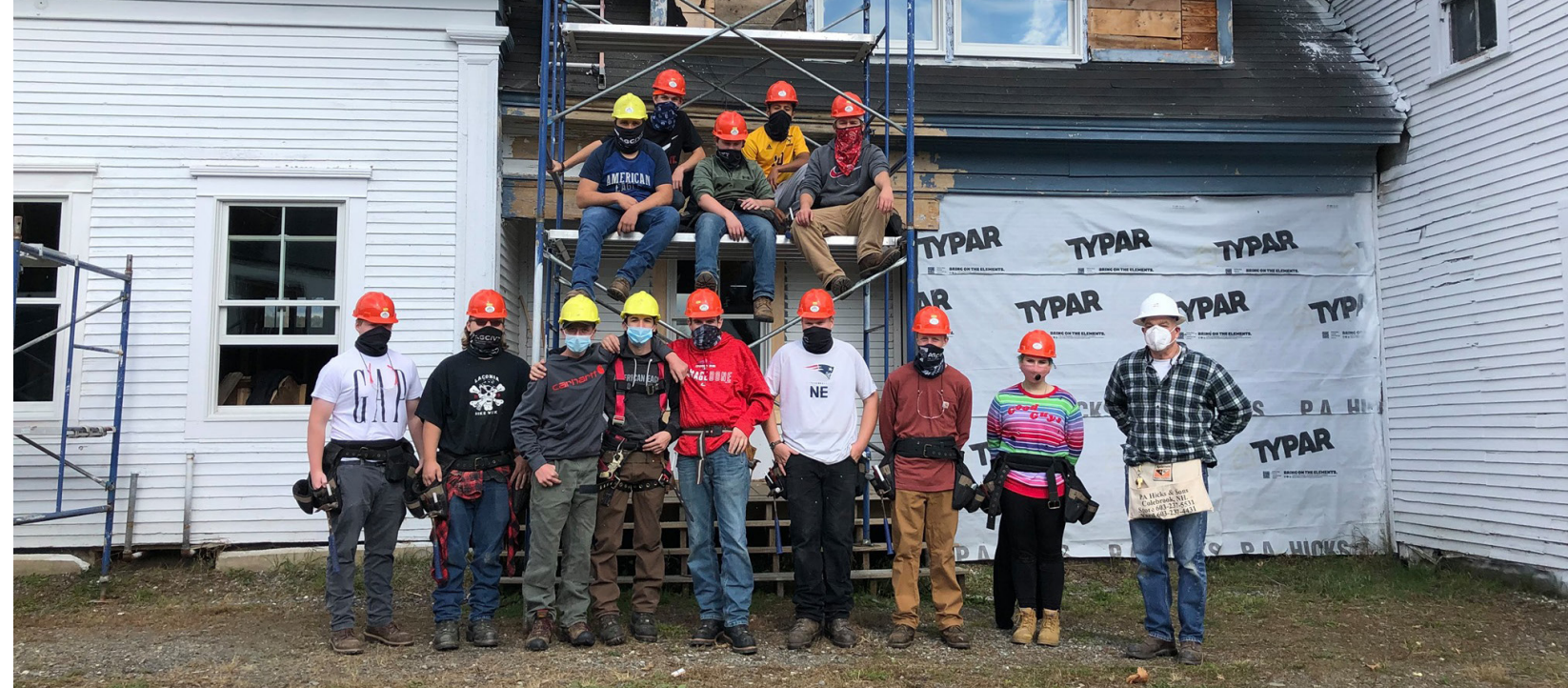
Canaan Memorial High School Building Construction and Restoration Carpentry program, Colebrook, NH. Photo: New Hampshire Preservation Alliance
