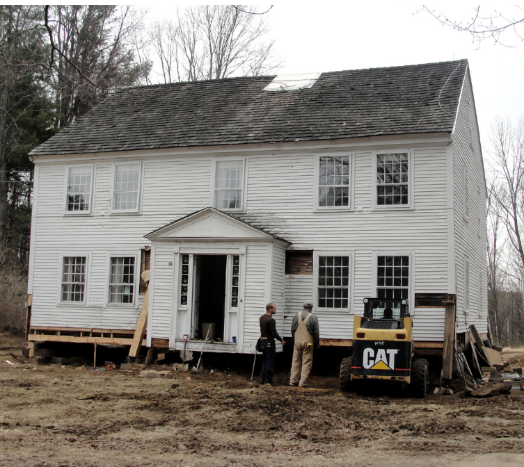
Foundation and sill work. Photo: New Hampshire Preservation Alliance
