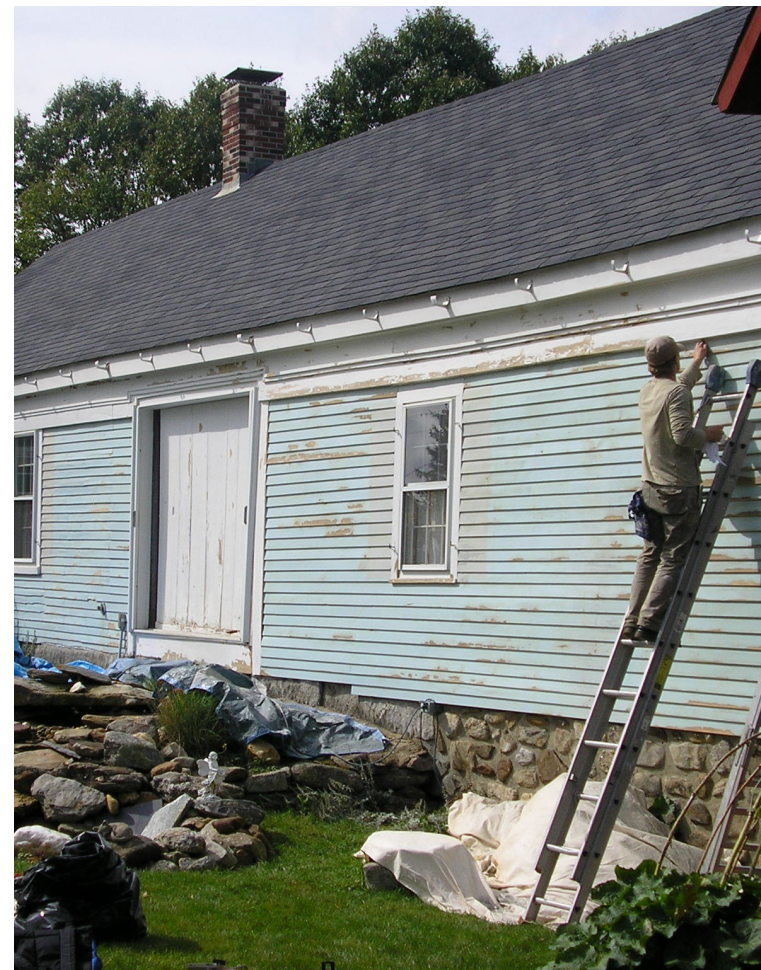
Painting work underway. Photo: New Hampshire Preservation Alliance
