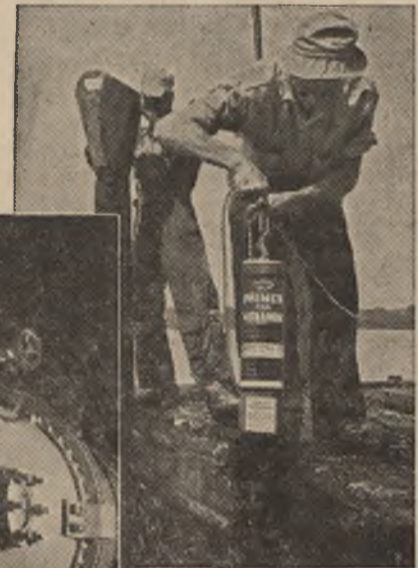
A. L. St. Peter, Princeton '37, supervisor blasting operation Susquehanna River Project, lowers a 5 1/2 inch "Nitramon" Primer into one of 600 drill holes preparatory to blasting a pipe line ditch.
