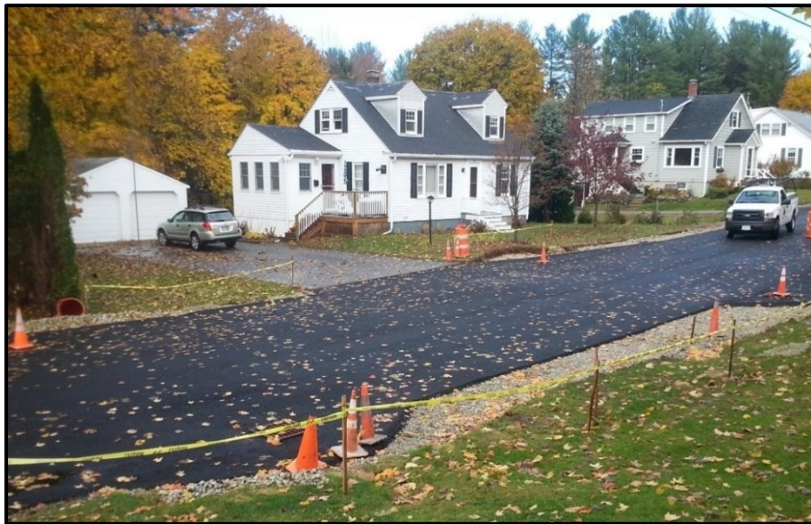
Figure 3: Post-construction picture of Grove St subsurface gravel filter, Dover, NH
