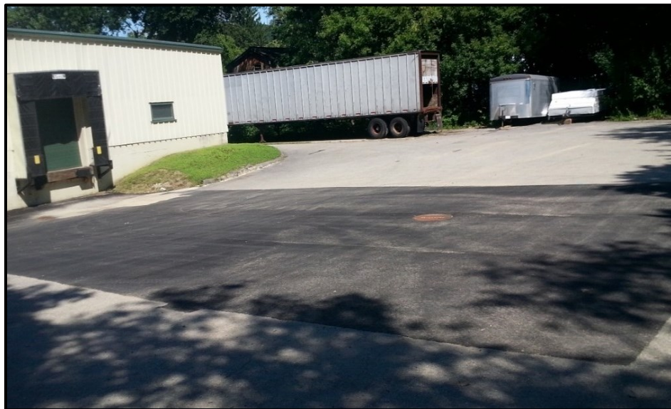
Figure 4: Post-construction picture of Kettlebell subsurface gravel filter, Dover, NH
