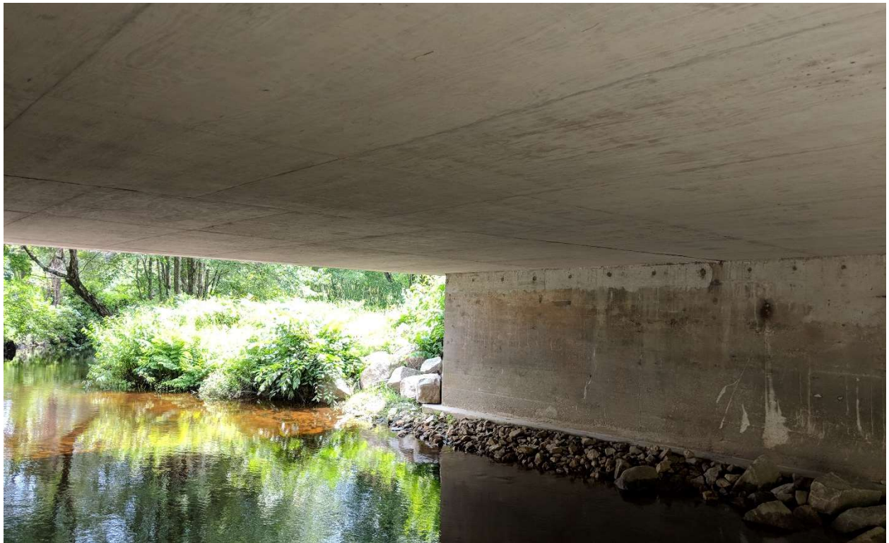
Figure 20: Concrete slab bridge structure example in Alexandria, NH.
