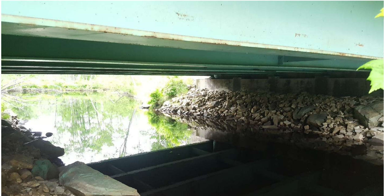
Figure 21: Steel I-beam with concrete deck bridge structure example in Wakefield, NH.
