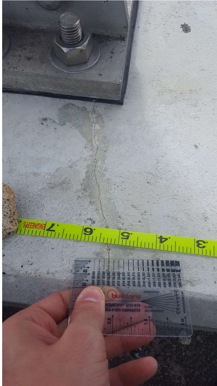
Figure 9: Crack comparator used to aid in crack width determination.
