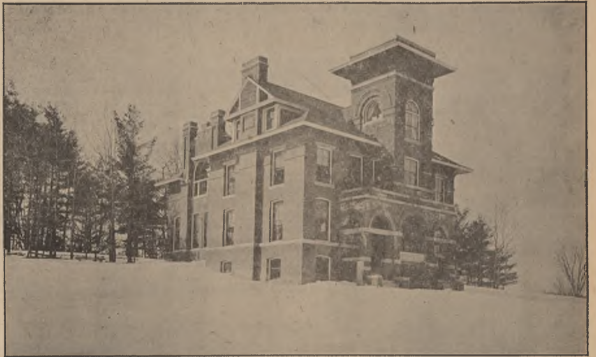
Old Nesmith as it looked before its first remodeling. Contrast this with Nesmith today.
