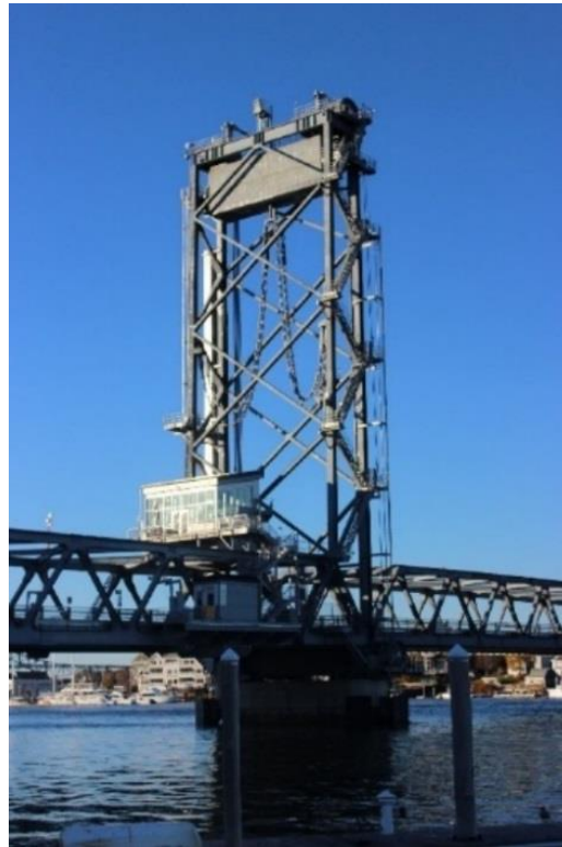
Figure 6 - Memorial Bridge (Portsmouth, NH) southern tower and counterweight
