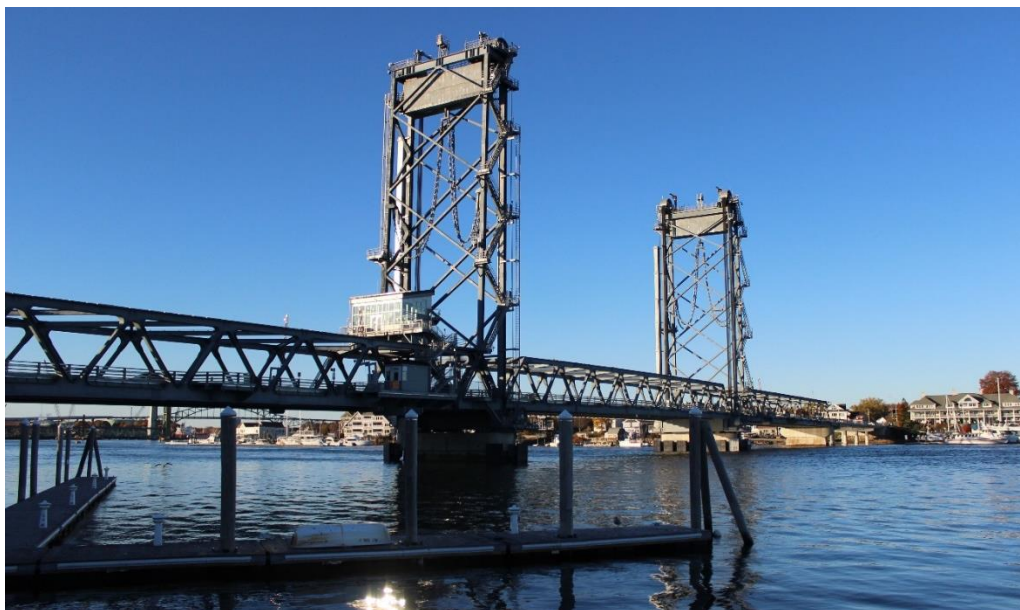
Figure 8 - The Memorial Bridge as seen from Portsmouth (2016)
