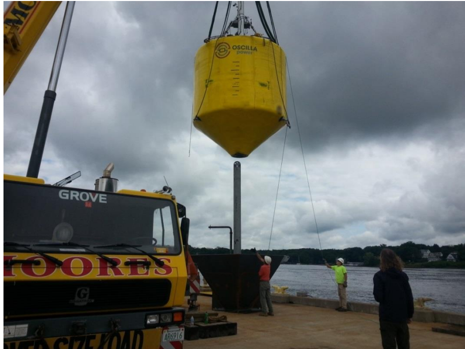
Figure 56: Buoy being mated to the heave plate.
