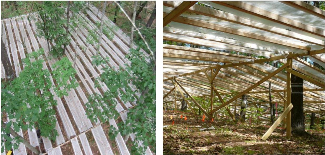
Figure 2. Aerial (left) and ground (right) view of throughfall removal structure simulating once in a century drought on mature trees at Thompson Farm, NH, U.S.
