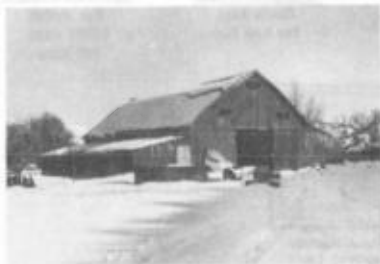
Before Renovation (Photo: Adrian Allen)
