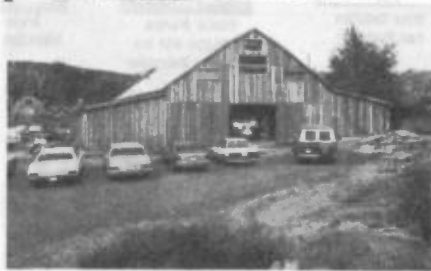
Finally— Completed (Photo: Adrian Allen)
