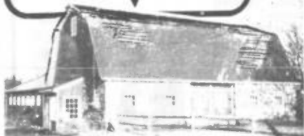
HAYLOFT STEPPERS BARN Sturbridge, Massachusetts
