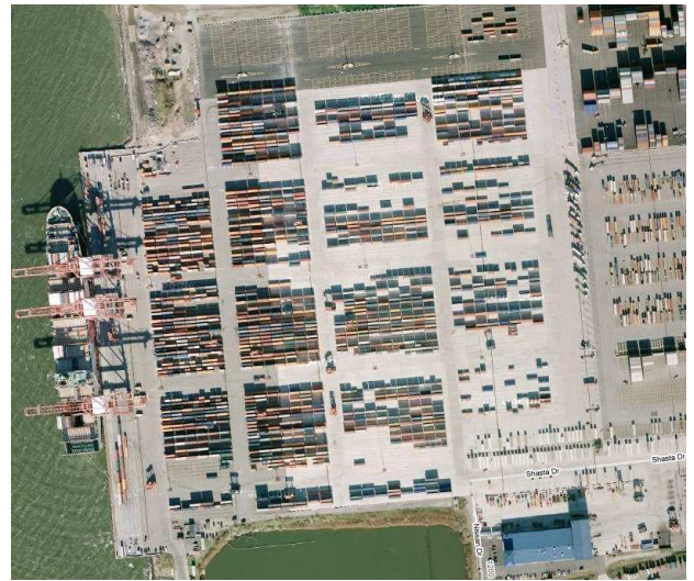
Figure 15: Aerial photograph of the zone 4.5 (source: Google Maps/Digital Globe) showing the container terminal characterized in Figure 10 and 14.
