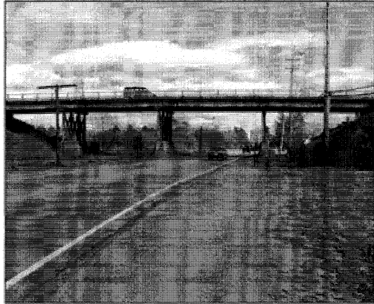
Figure 3: Rollins Road Bridge prior to new bridge construction (Bowman M. M., 2002)
