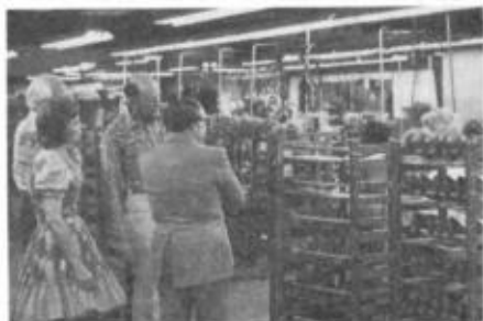
Chuck LeMons demonstrates the toe-forming operation in the Lasting Room. Then Don demonstrates how heels are attached with an automatic five-nail machine, to Cal, Virginia, Randolph, Karla, and Stan. The final shots below are in the Packing Room.
