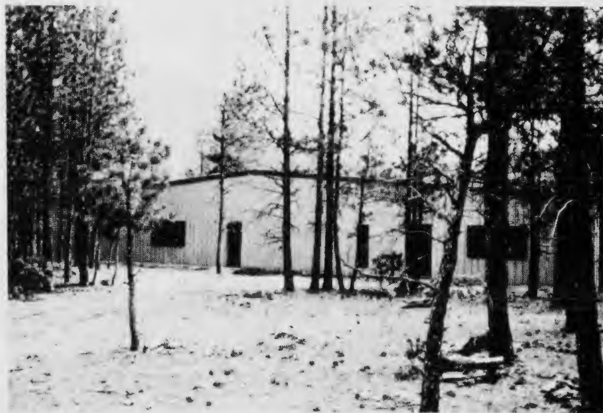
Viewed from the highway is the recently completed square and round dance center near Missoula, Montana, planned and built by Ray and Afton Granger. The building houses a dance hall (on the left), apparel shop and eating area (on the right), and offers a vista of pine covered mountains.
