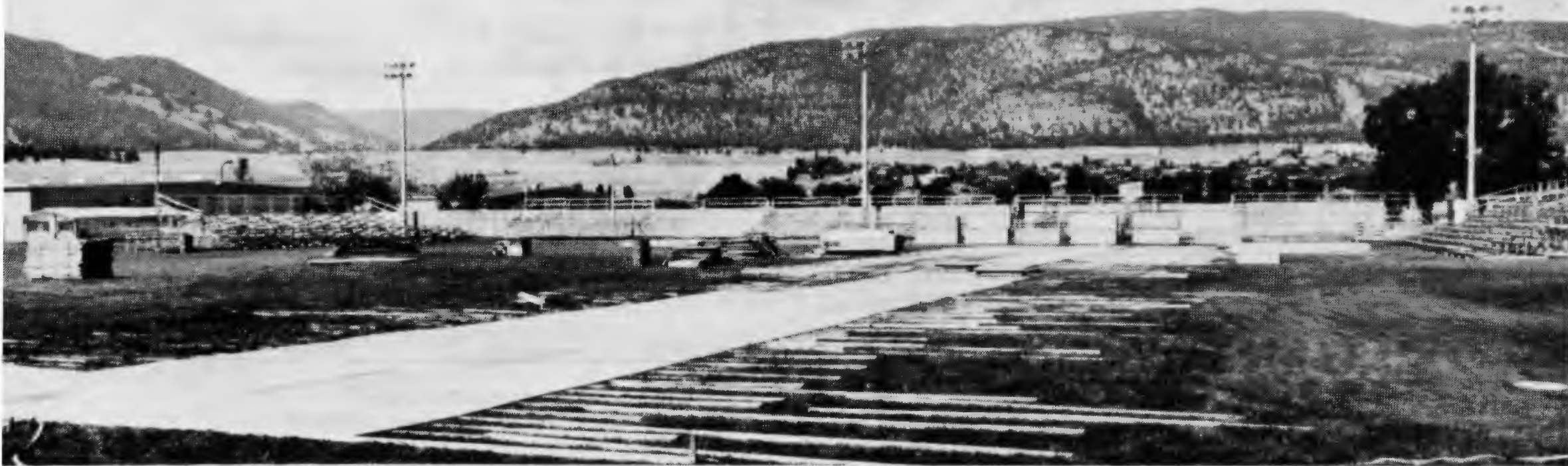
THE BEGINNING — 2" x 4" stringers are laid out on the lawn of King's Park.
