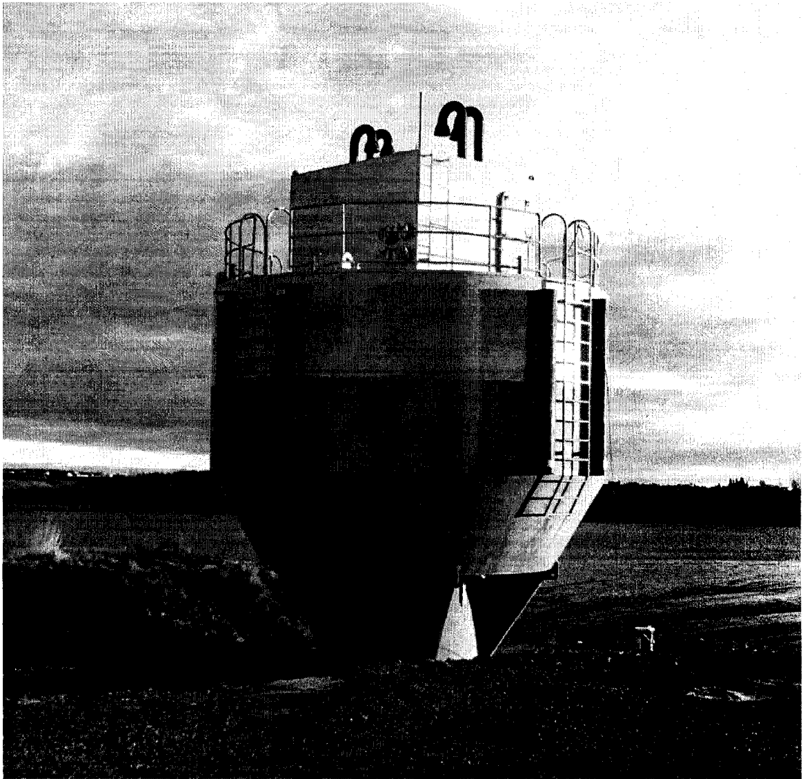
Figure 7.12: Assembled 20-ton buoy at final construction site in Hillsborough, NB, Canada.
