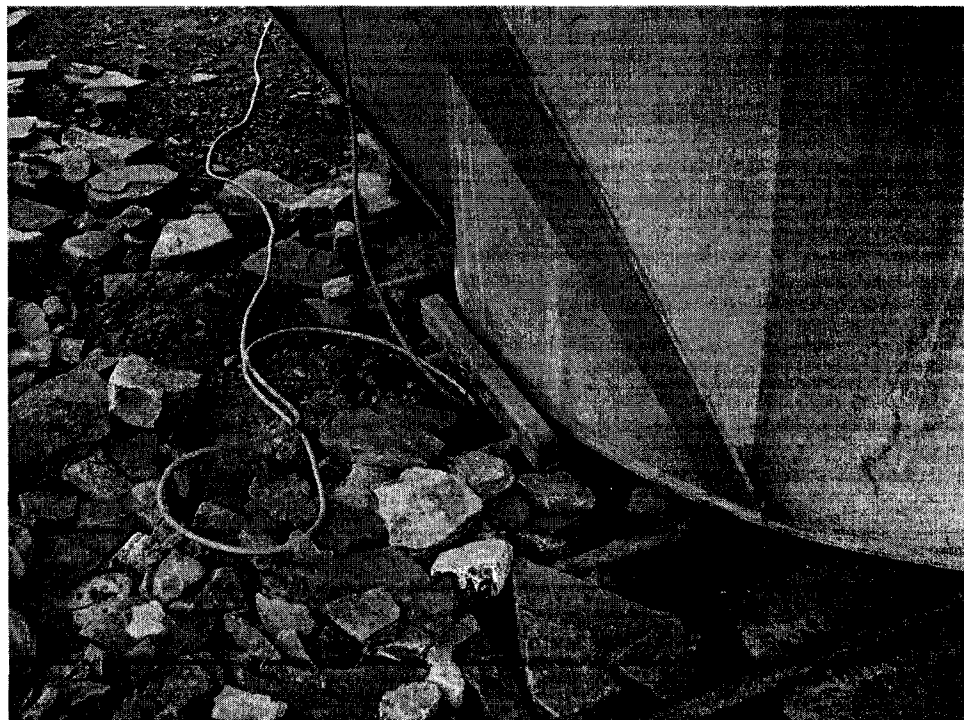
Figure 7.9: Close up of steel rods placed under buoy to allow the buoy to roll into the ocean during launch.
