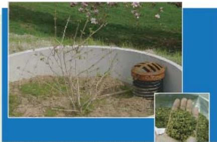
Bottomless tree box filter after installation (left). Close-up of the coarse sand-compost media used in the tree box filter. The 76% coarse sand/24% compost mixture has 10% organic matter and infiltrates water at a rate of 14.6 inches/hour in the laboratory (right).
