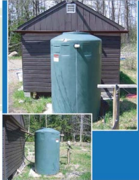
550 gallon cistern installation collecting rainfall runoff from a guttered roof.
