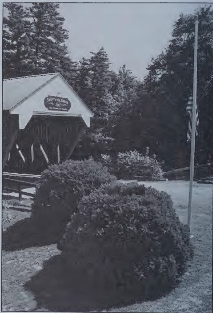
Swift River Bridge
