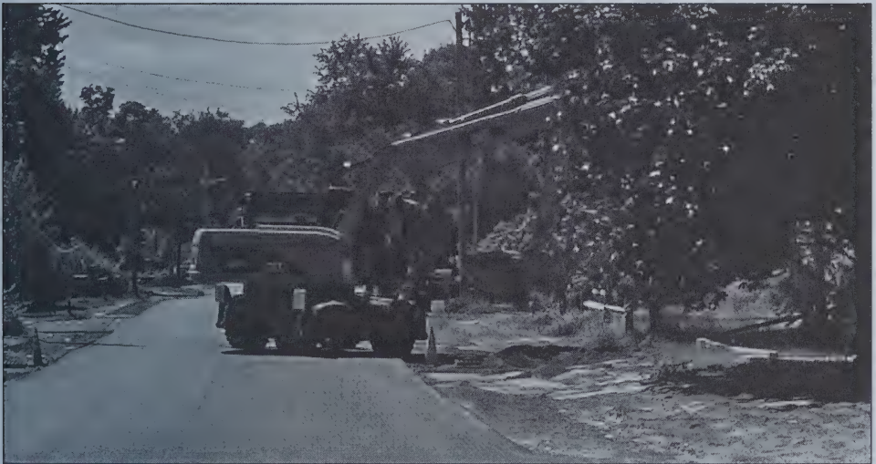
Infrastructure Road Improvements on Valley View Road, North Conway Village
