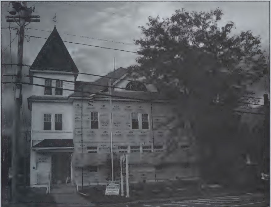
Town Hall Renovations
