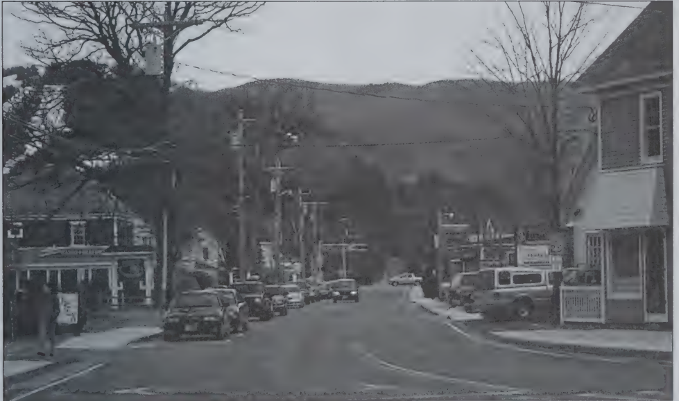
Seavey Street Reconstruction
