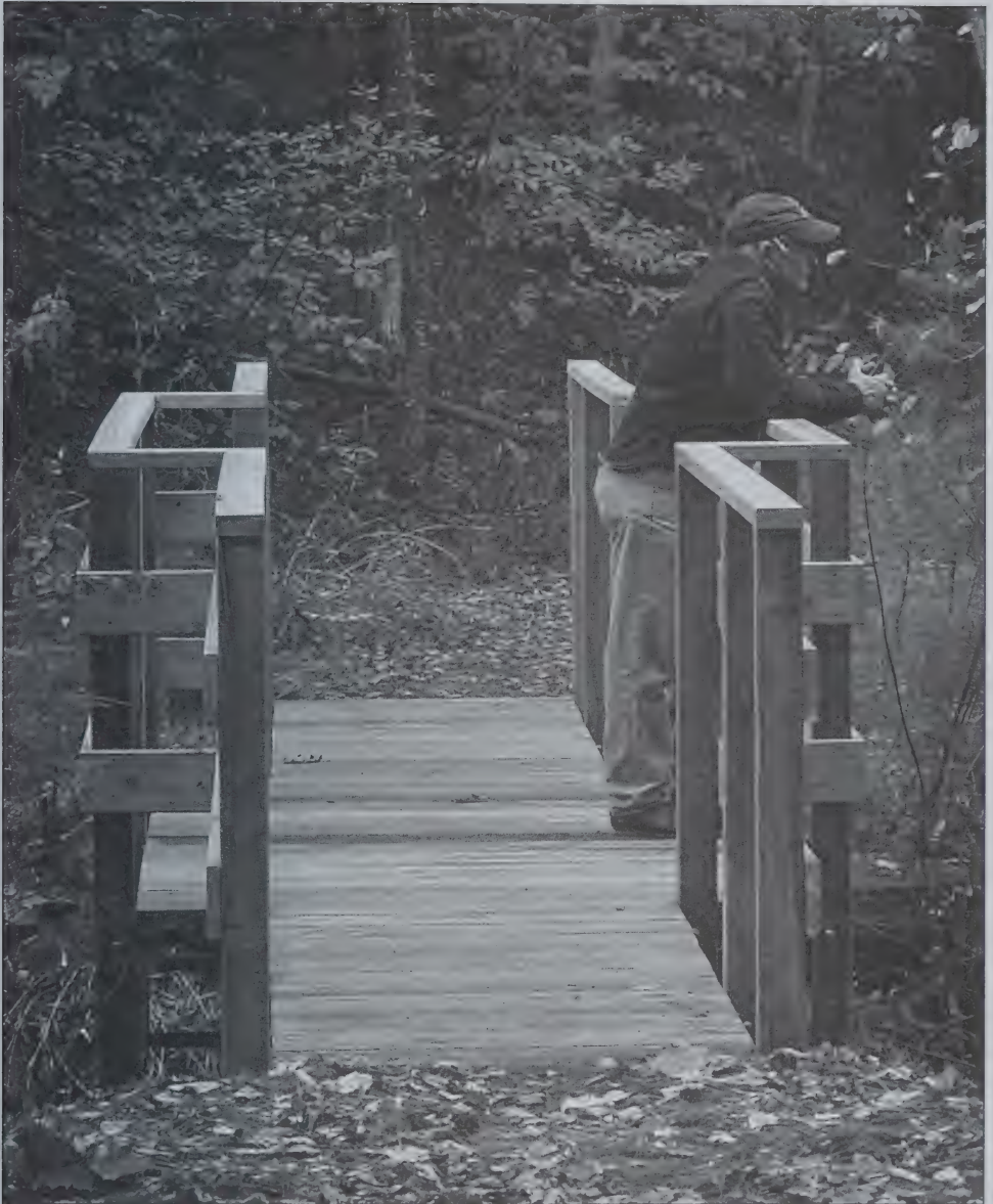
PUDDIN' POND RECREATION TRAIL BRIDGE TOWN OF CONWAY CONSERVATION LAND
