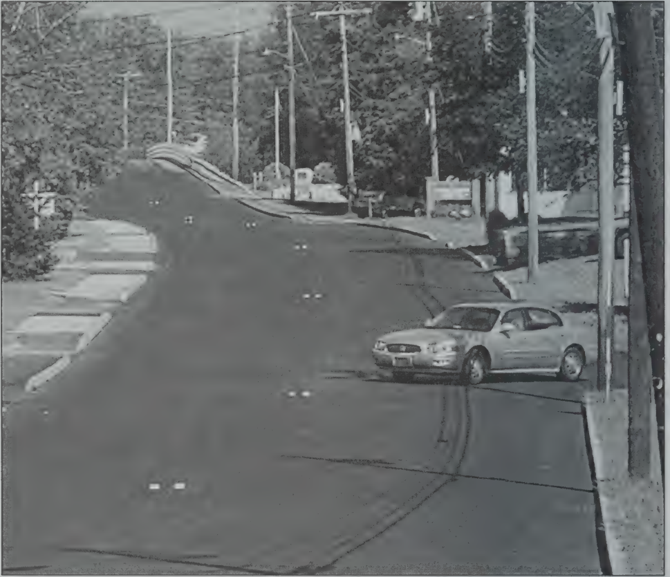
West Side Road Reconstruction
