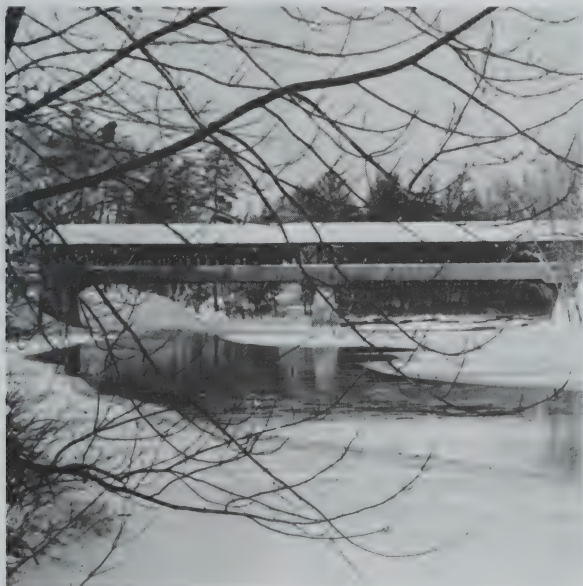
Saco River Covered Bridge
