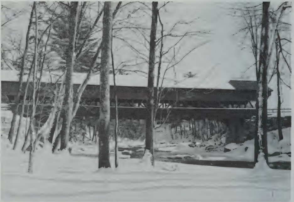
Saco River Covered Bridge
