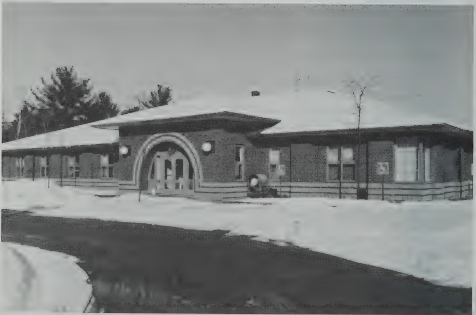
Conway Police Station
