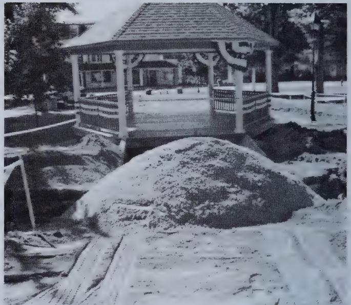
Right: The first of 65 tons of crushed glass used as aggregate instead of gravel for the new sidewalk that the Parks Department prepared for what is now a very nice sidewalk and handy capped excisable toe the community park band stand.
