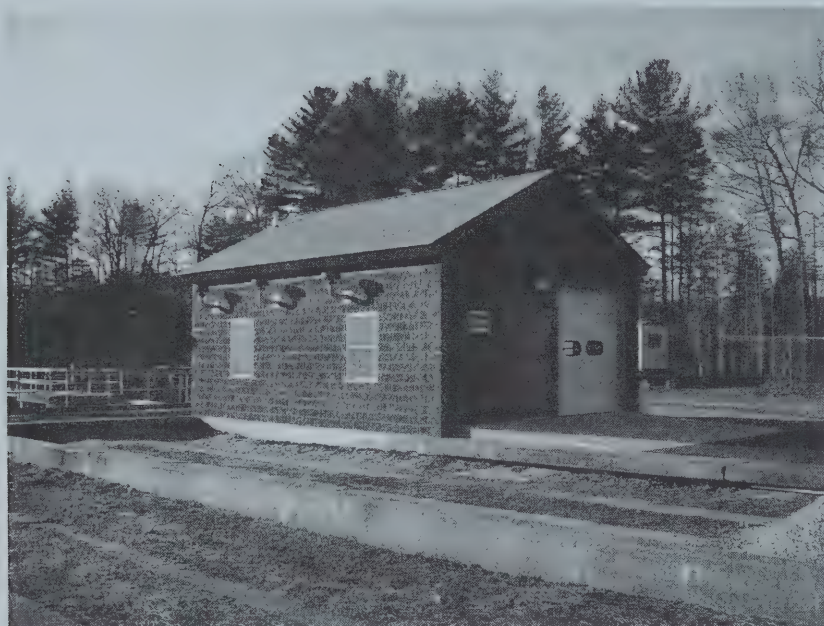
The new blower building. Photo courtesy of Ken Levesque.
