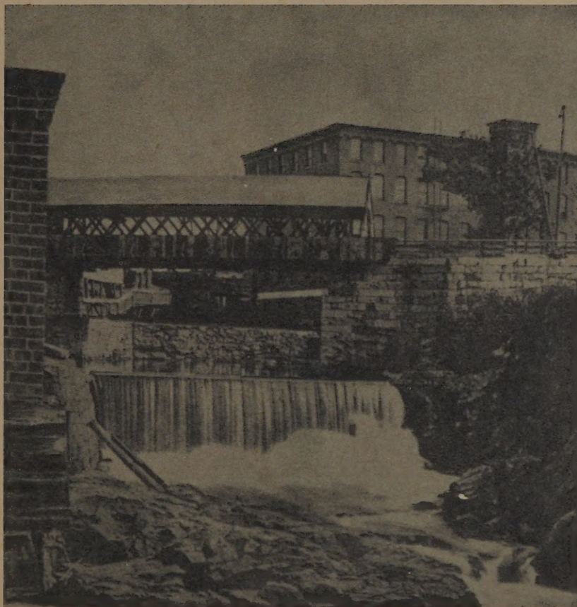
Pembroke Hill Dam, Main St. Bridge and Part of Webster Mill, Suncook, NH
