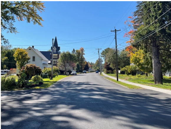
Newly paved South Winchester Street
