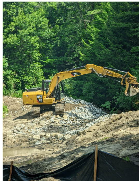
Work being done at Old Richmond Fire Pond
