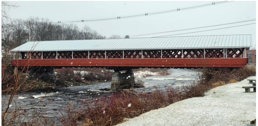
Newly painted Thompson Covered Bridge
