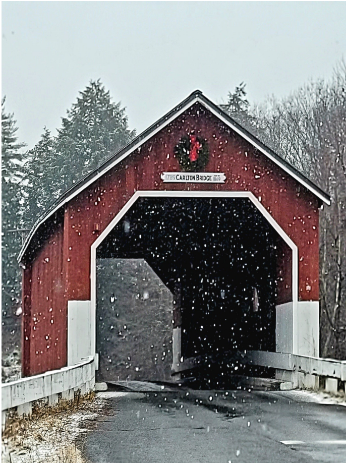
Carlton Covered Bridge in the winter
