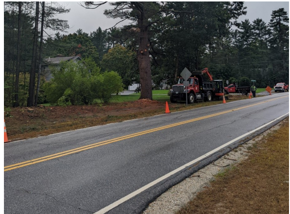
Sawyers Crossing Road
