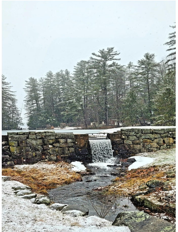
Swanzey Lake Dam in the winter
