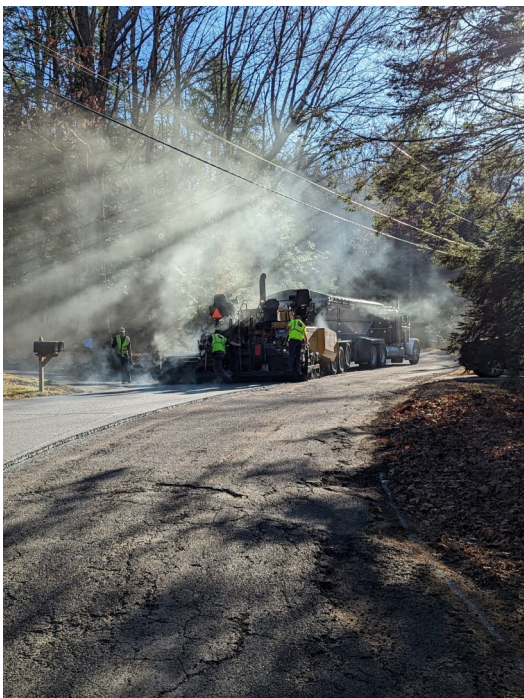
Paving of Foxglove Lane
