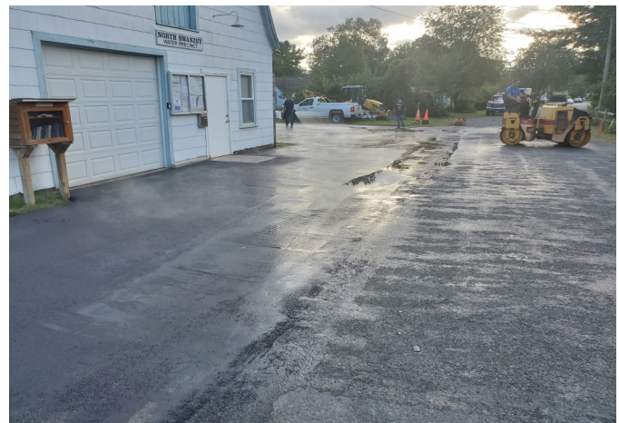
Public Works Department work on an apron and paving the driveway at the North Swanzey Water and Fire Precinct
