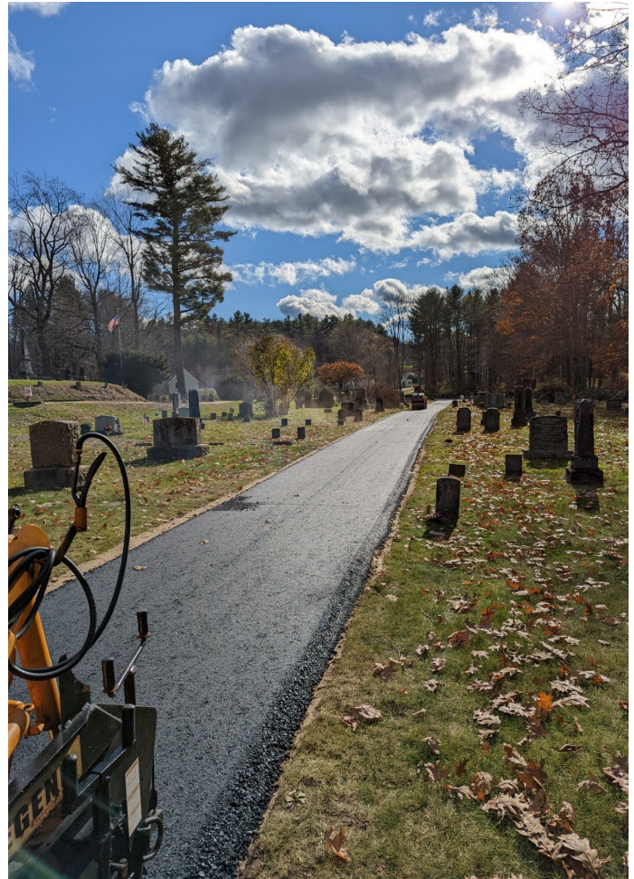
Oak Hill Cemerty Paving
