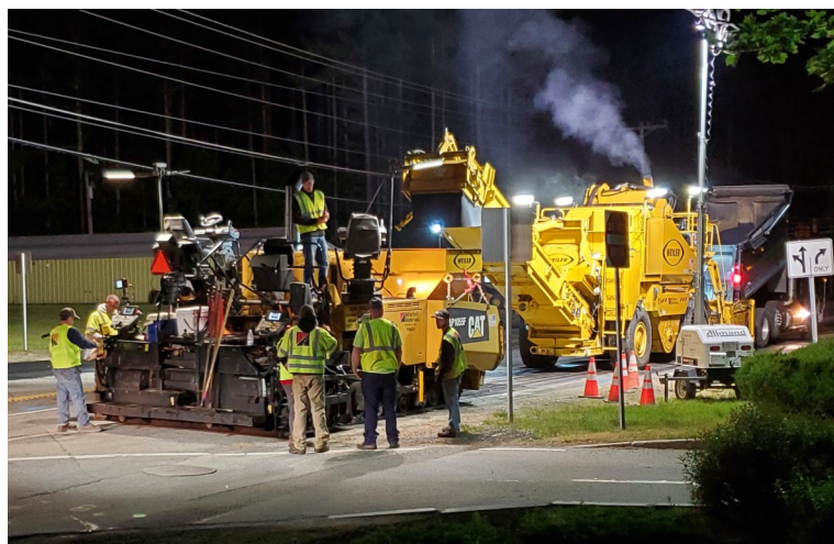
Paving on Route 10
