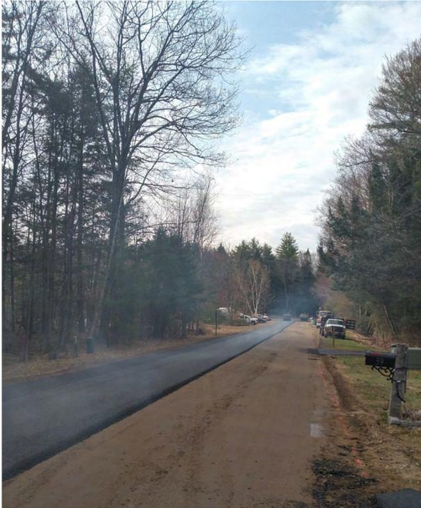
Road paving plans for 2022 are to finish the final wearing course on Ann Lane, Hooke Road, Deer Run, Kelsey Drive and Kirstens Landing. These 5 roads will be done first. Remaining funds from the budget line for Hot Top and Reconstruction Materials will be used for Phase 2 of Whittier Drive started in 2017, with 1 more mile to rebuild. This road is over 30 years old and in very poor condition.
