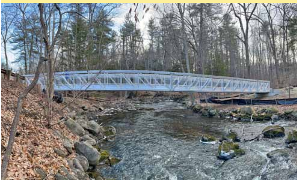
AFTER A YEAR OF WORK AND WITH THE SUPPORT OF ALMOST 400 DONORS, THE NEW KENNY ROTNER FOOTBRIDGE WAS INSTALLED IN JANUARY 2021. THE 100' ALUMINUM SPAN LINKS THOMPSON LANE AND STEVENS WOODS ACROSS THE FRESHWATER PORTION OF THE OYSTER RIVER. NOW THE ORCHARD DRIVE NEIGHBORHOOD IS WITHIN QUICK WALKING DISTANCE OF DURHAM'S CENTER, AND THE NETWORK OF BEAUTIFUL, FORESTED TRAILS EXTENDING TO DURHAM'S DOE FARM CAN BE EASILY REACHED FROM TOWN ON FOOT. Courtesy DPW
