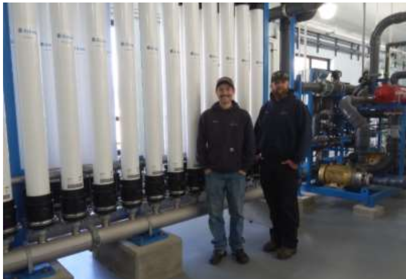
Dylan and Wyatt at the Water Treatment Plant
