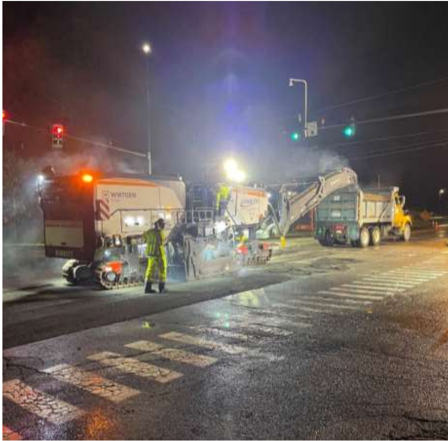
Milling at the Lyme Road and Park Street Intersection
