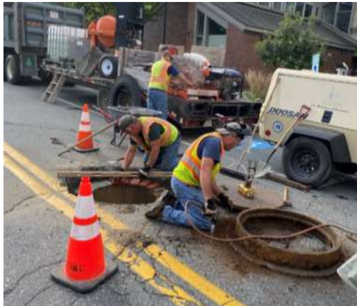
Manhole Repair on South Street
