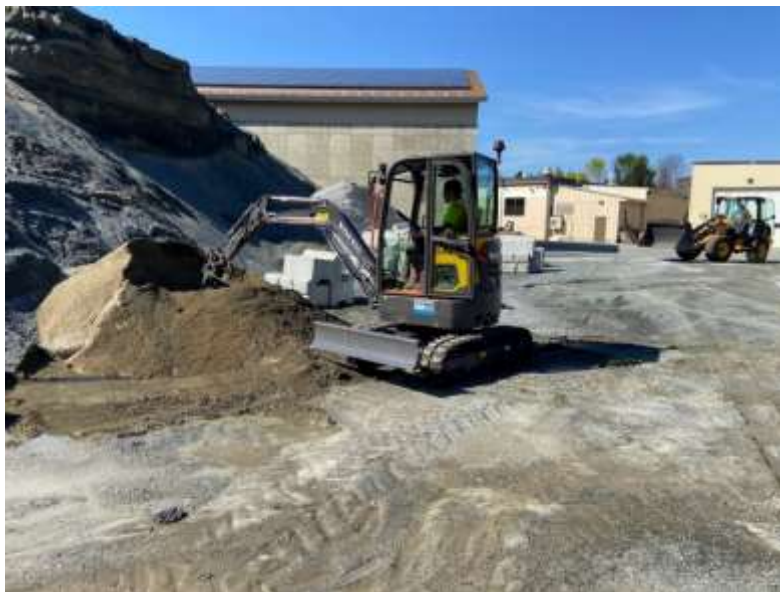
Staff Trying out an Electric Excavator
