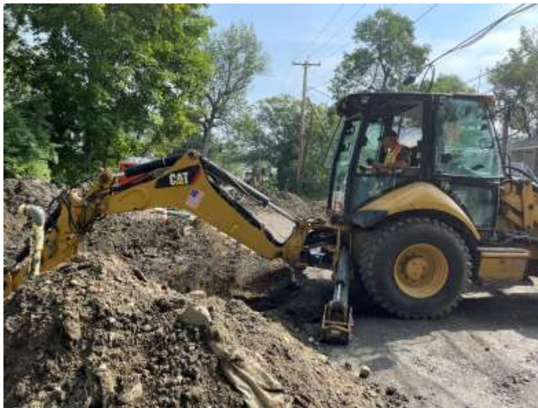
Jim Excavating for the New Water Line on Summer Street
