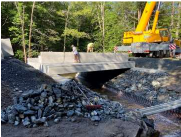
Setting bridge deck at Ruddsboro & Three Mile Roads
