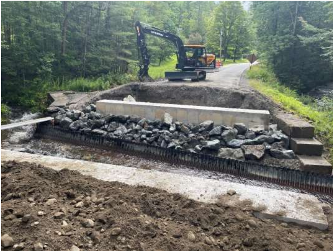
New Footings for the Ruddsboro Road Bridge
