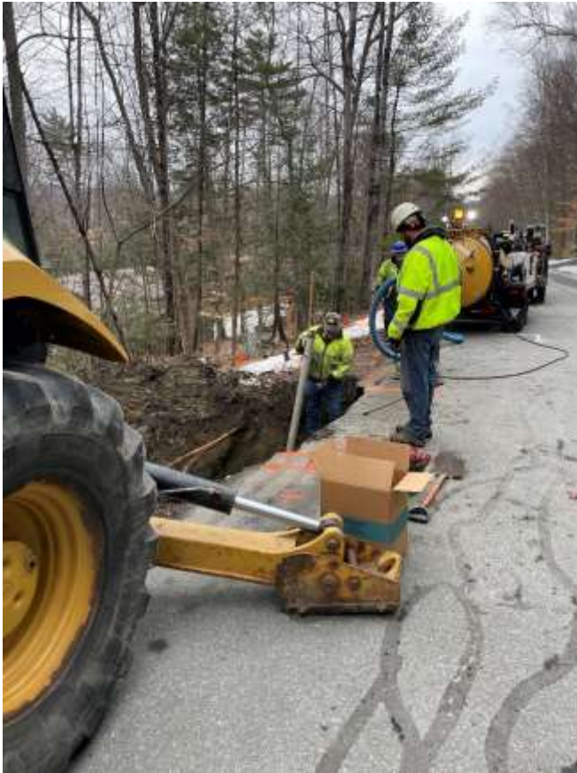
Fixing a Broken Water Main on Low Road
