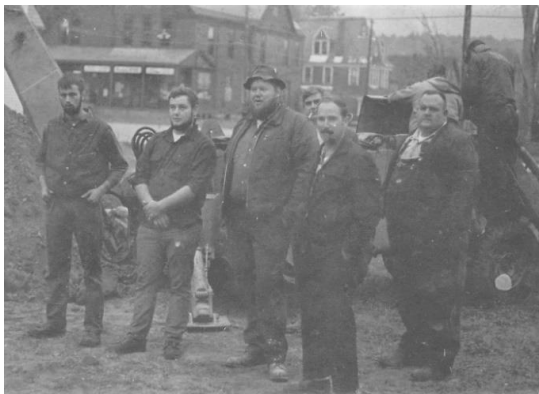
Groundbreaking for New Fire Station – 1973
