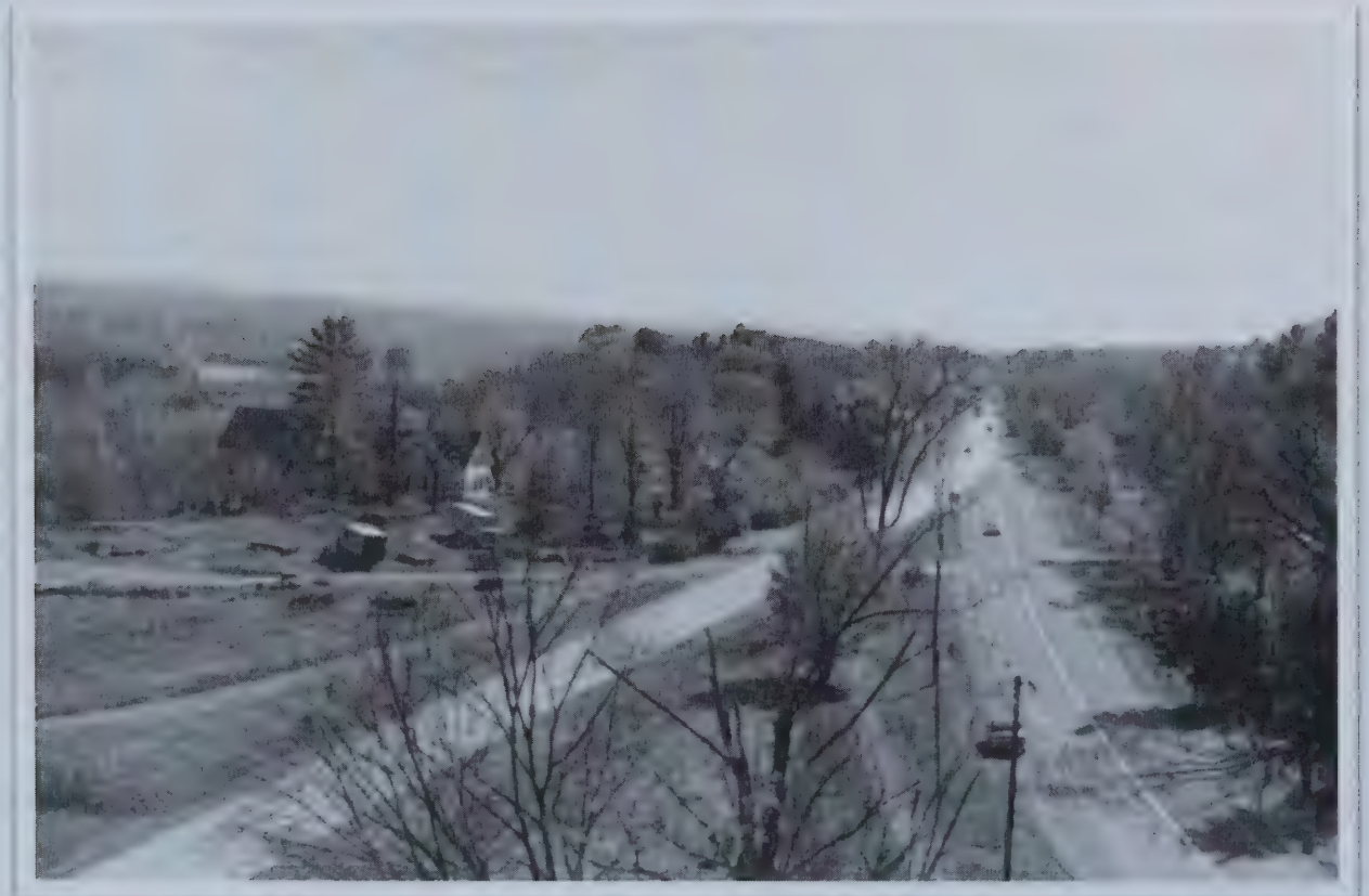
Undated photo of the Route 3 & 4 junction taken from the Congregational Church steeple
