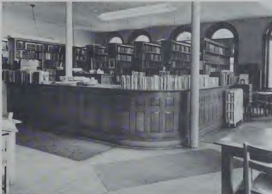
Library reading room in Chandler building leveled by urban renewal.
