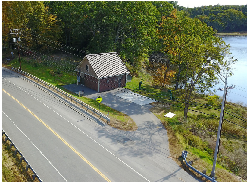
Dover Road/Route 108 Pump Station. At the March 12, 2019 Town Election, Durham residents will be asked to vote on a referendum question on the Warrant to authorize the bonding of $2,680,000 for the construction of a new force sewer main which will run from the pump station to the Wastewater Treatment Plant. Courtesy DCAT Studios
