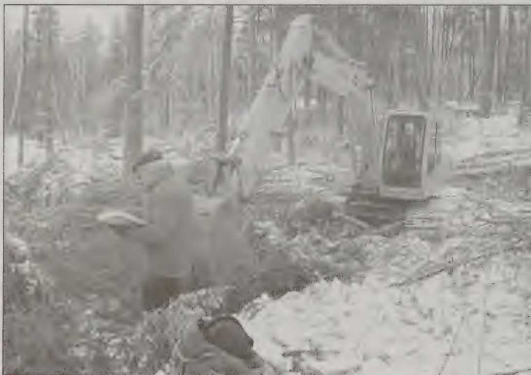
Don Bent oversees test pit excavation.
