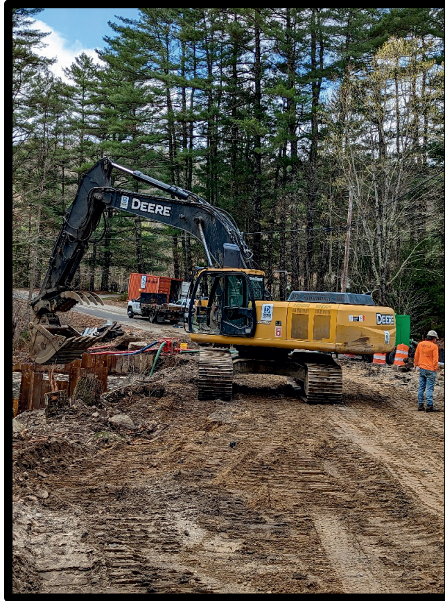
Photo of White Plains Bridge under construction
