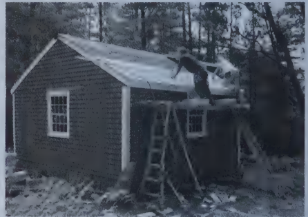
Frank Baker and Brad Hartwell re-shingle the roof of the Tucker Mountain Schoolhouse.
