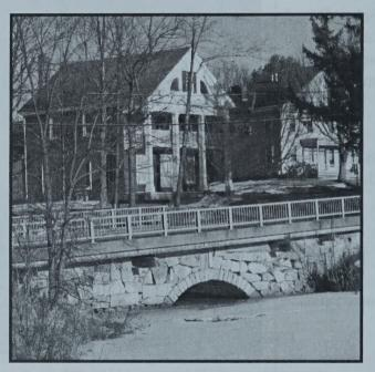
The bridge on South Main Street over the outlet of Village Pond dates from 1835 when the stone arch was built by the Town of Troy. The original, filled spandrel, split stone arch structure remains visible on the upstream (west) side of the bridge.
