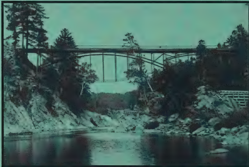
The old "Pumpkin Seed" Bridge constructed in 1886
